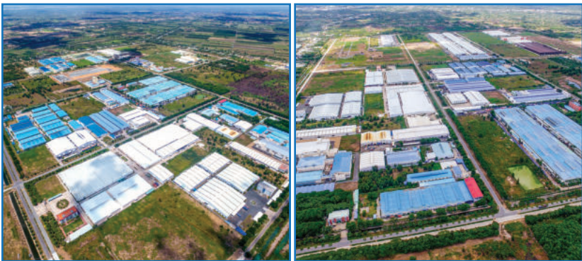
1.5. Long Giang Industrial Park
